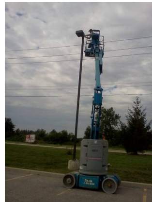
One of our workmen fixing the parking lot lights.
